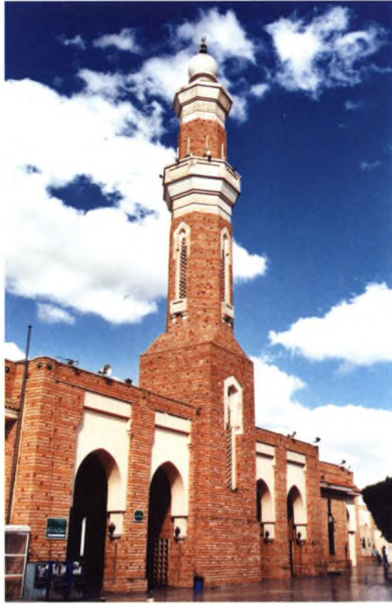
Minaret of the mosque of Ibn Abbas in At-Ta'if
